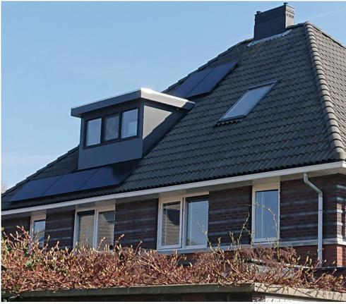
The northwest side of the roof has five modules with one pop-out and one skylight to design around.
