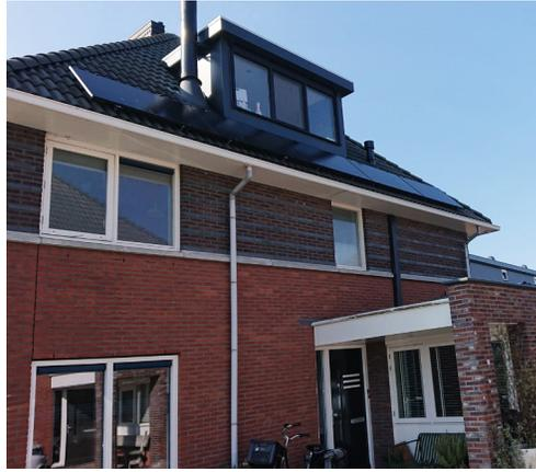
The northeast side of the roof has six modules below a pop-out and multiple roof obstructions
